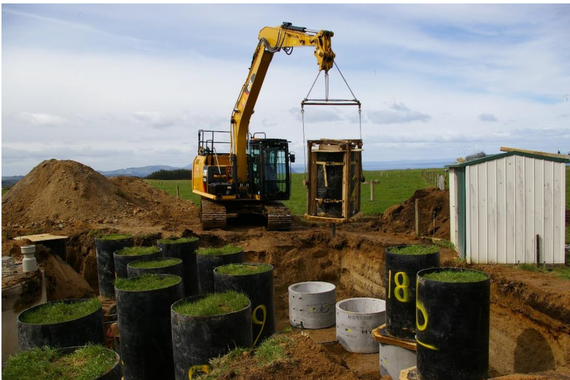
Figure 2. Lysimeter facility at Tihoi under refurbishment. Note the grey dropper pipe under the lysimeter housing the fibreglass wicks.
